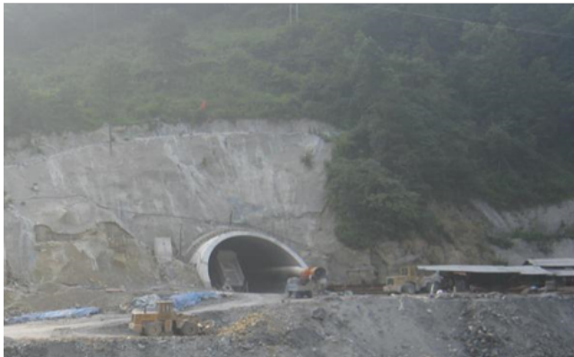
Fig. 1 The left tunnel entrance
