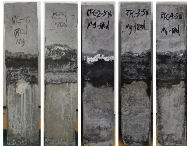
Figure 6: Corrosion morphology of RPC in \text{MgSO}_4 solution Note: The replacement rate is 0%, 10%, 20%, 30%, and 40% from left to right.
