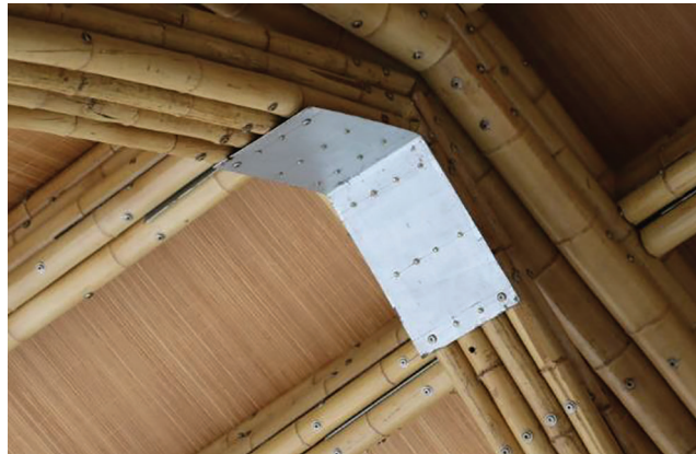
Figure 2: Bamboo structure with bolted connections
