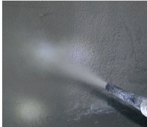
Figure 9: Typical shotcrete spray
