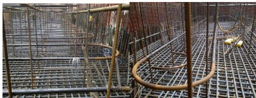
Figure 4. Field cooling piping layout.
