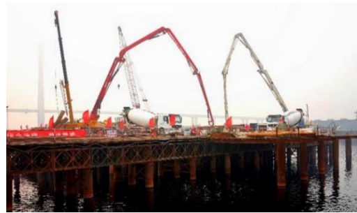
Figure 2. Construction of 2# pier bearing platform for Haihe special bridge.
