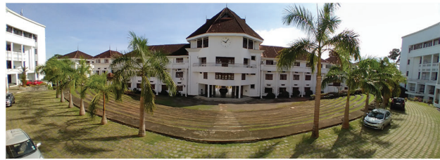
Figure 2: Panoramic imagery of SAINTGITS AMPHI–The Arc-shaped twelve stair iconic Amphitheatre: View from the first floor of Centre Lecture Complex (CLC)
