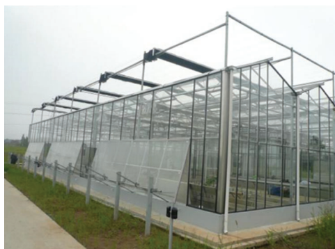
Figure 1: Exterior view of venlo glass greenhouse in Nanjing, China. The greenhouse structure has an area of 30 m in length × 9.6 m in width, 4.5 m in height with north-south orientation
