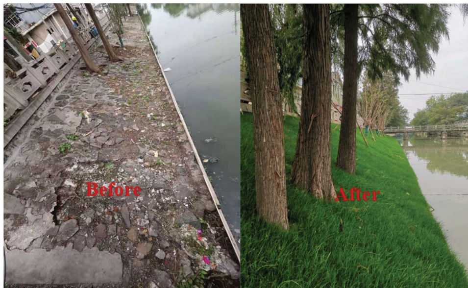
Figure 7: Application of PVC in ecological slope protection
