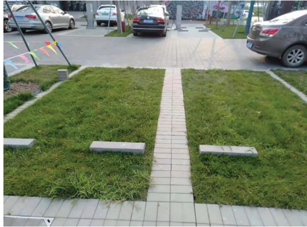
Figure 6: Ecological parking space
