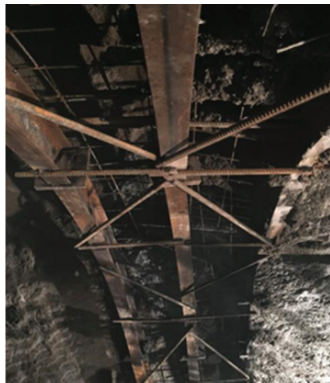
Figure 6: The connecting steel bars
