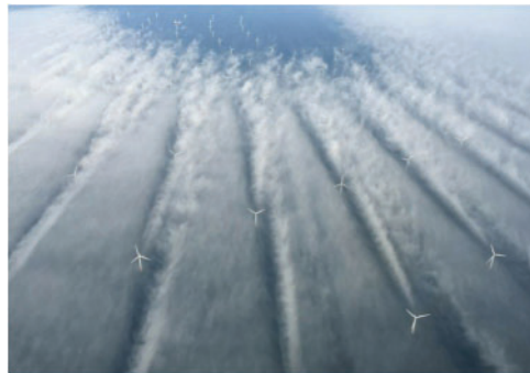
Figure 1: Horns Rev II offshore wind farm in Denmark [8]
