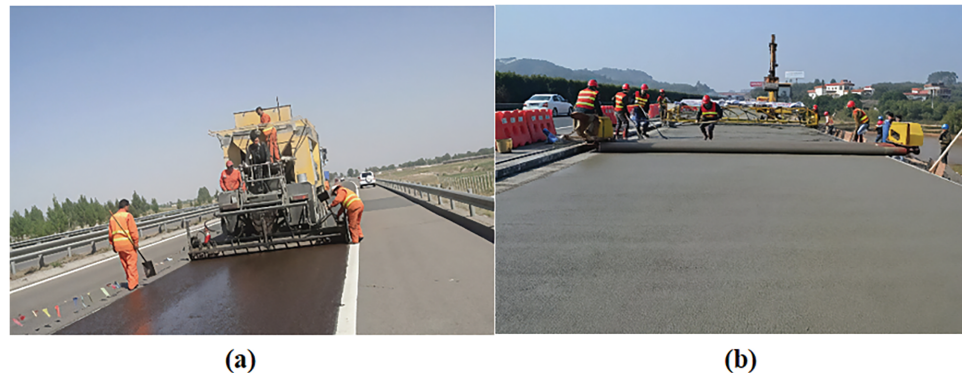
Figure 1: (a) Schematic diagram of ultra-high performance fiber-reinforced concrete bridge deck pavement structure and (b) Compaction diagram for ultra-high performance fiber-reinforced concrete surface layer in bridge engineering
