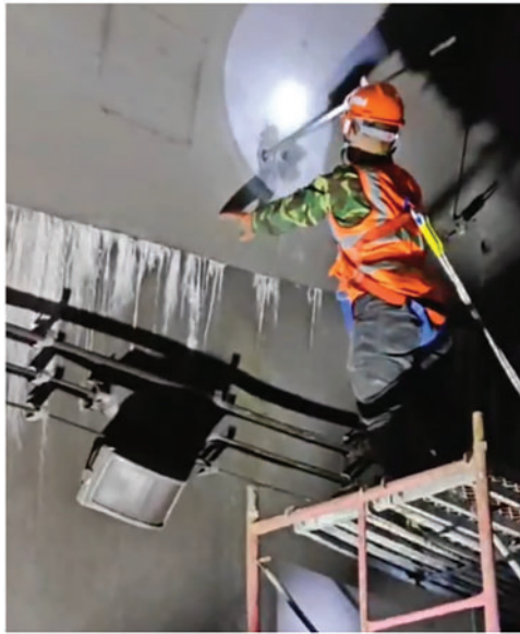
Figure 19: A core sampling at the tunnel arch waist
