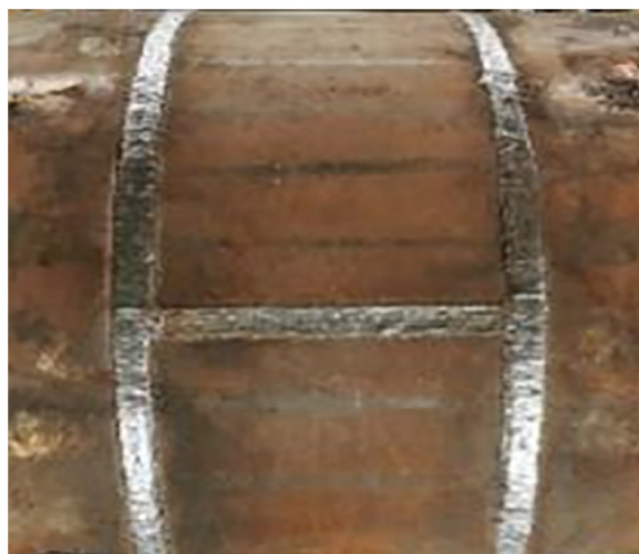
Figure 4: Splicing weld
