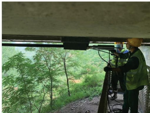
(a) Installation process
