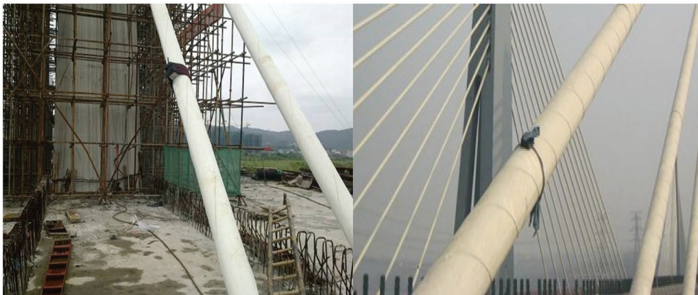
Figure 10: Photos of cable tension monitoring
