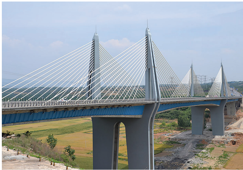
Figure 1: Photo of the bridge
