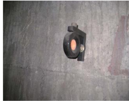
Figure 7: The installation of reflection prisms of supervision points
