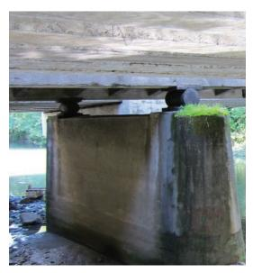
Figure 10a: Type of roller restraints used in older concrete bridges.
