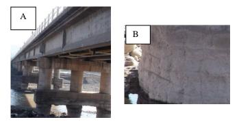
Figure 8: a) Totkabon Concrete Bridge b) Totkabon middle pier water scour.
