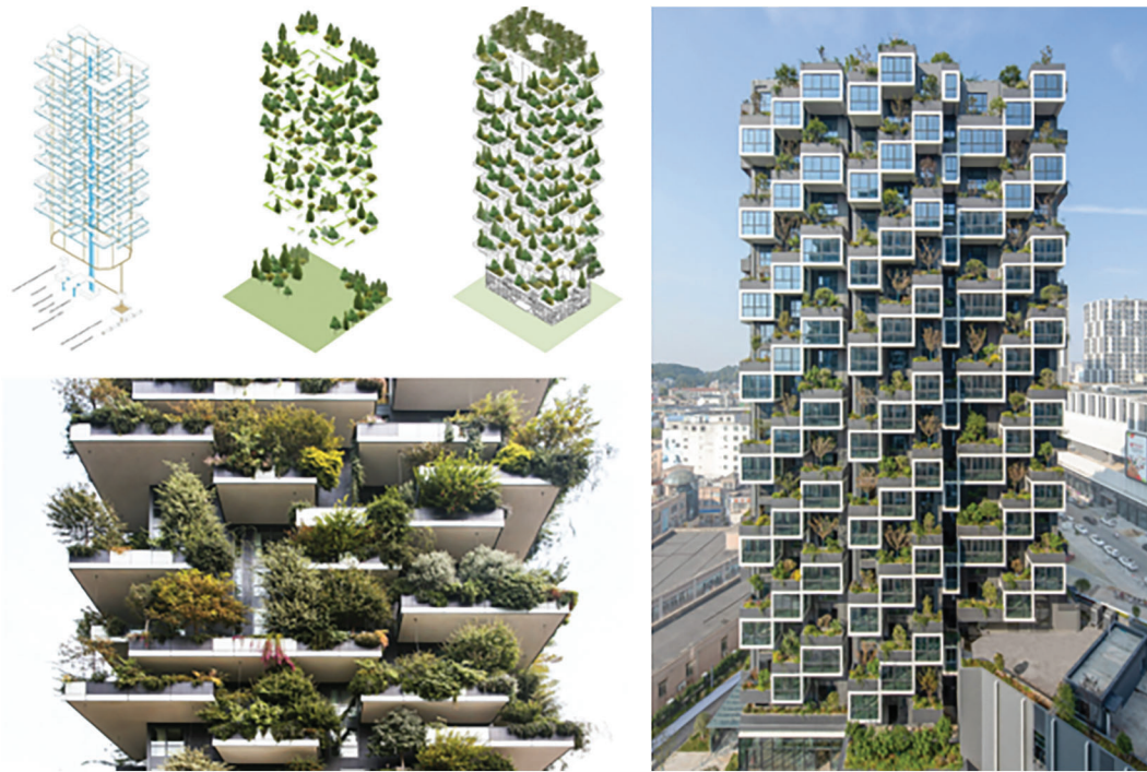
Figure 22: Image of the world's first vertical forest. Adapted with permission from References [138–140], Copyright © 2022 İklim Polat Interior Architecture. All rights reserved, 2024 ArchDaily. All rights reserved and 2022 Dezeen. All rights reserved
