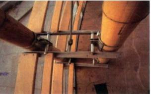
**Figure 20:** Connection between main structure and enclosure structure [34]
