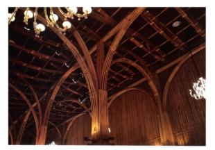
Figure 5: Lashing joint in Vietnam Pavilion [34]
