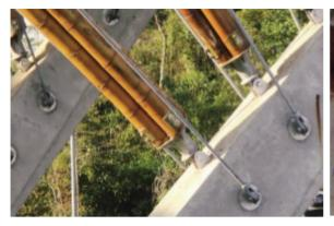
**Figure 19:** Connection between raw bamboo and concrete [50]
