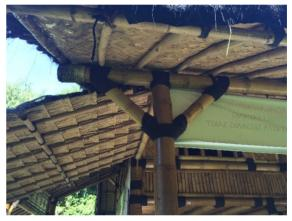
Figure 4: Lashing joint by palm rope
