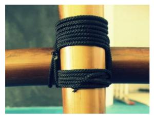
Figure 3: Lashing joint [33]
