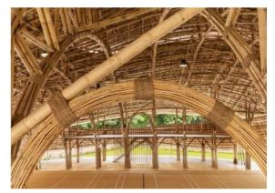
Figure 6: Lashing joint by hemp rope [35]
