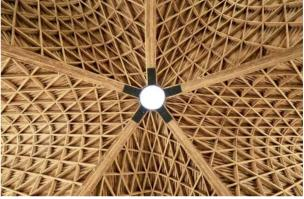
**Figure 22:** Steel member joint in Bamboo Luum Temple [51]
