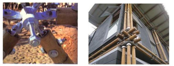
Figure 13: Common form of steel member joint [34] Figure 14: Multi-layer metal cage [44]
