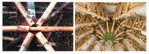
Figure 17: Simple steel plate joint [34]
