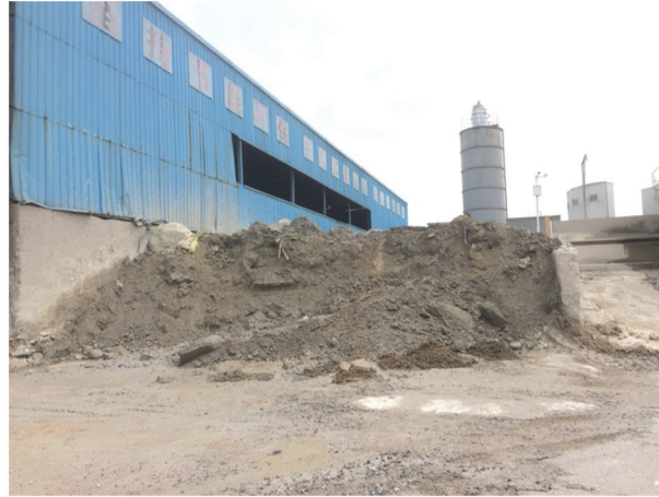
Figure 1: Waste residue of ready-mixed concrete station
