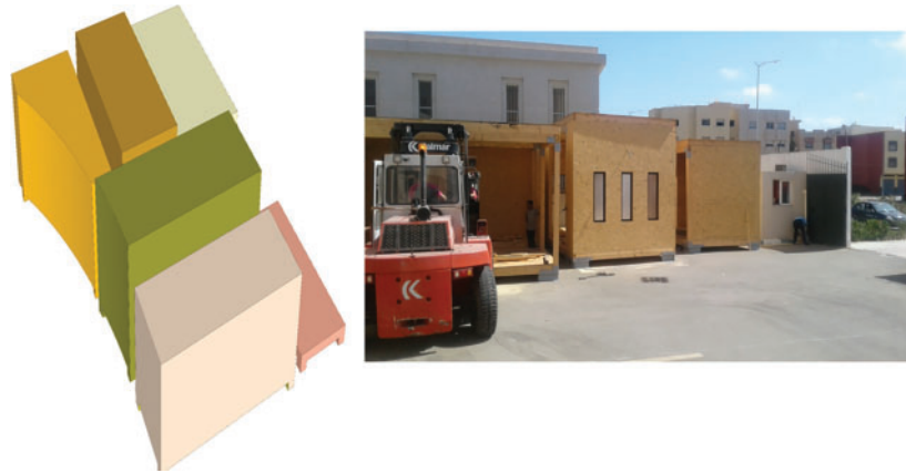
Figure 4: The different blocks of the A'freehome house
