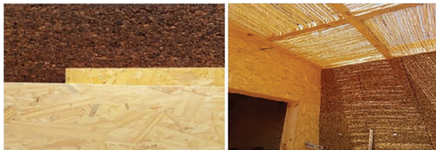
Figure 5: Oriented Strand Board (OSB) panel, Cork, and Reed used
