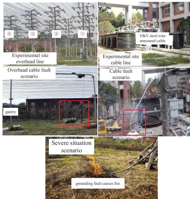
Figure 9: Real distribution network experiment site
