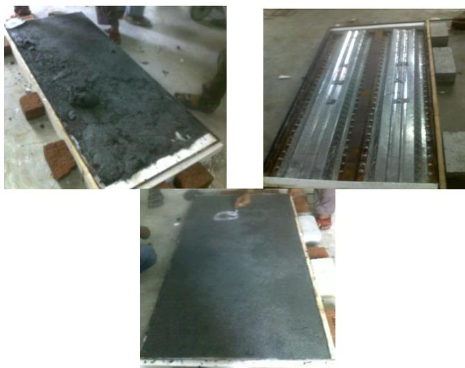
(a) Casting of bottom skin      (b) Connection of bottom skin and profiled sheet with self tapping screws      (c) Casting of top skin
