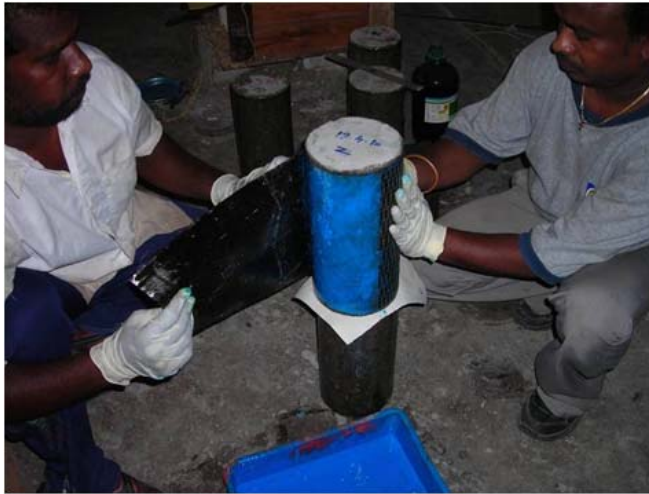
Figure 6: Wrapping of Cylinder with Carbon Fibre
