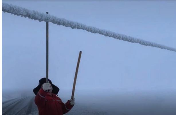
**Figure 1:** Manual inspection of ice-covered wires
