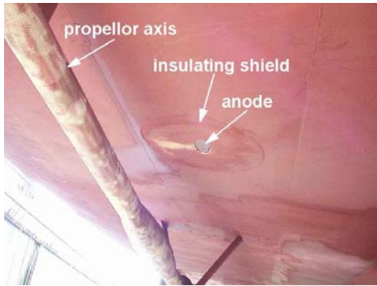
Fig. 11 : Part of a ship's surface for which ICCP is employed showing an electrode.
